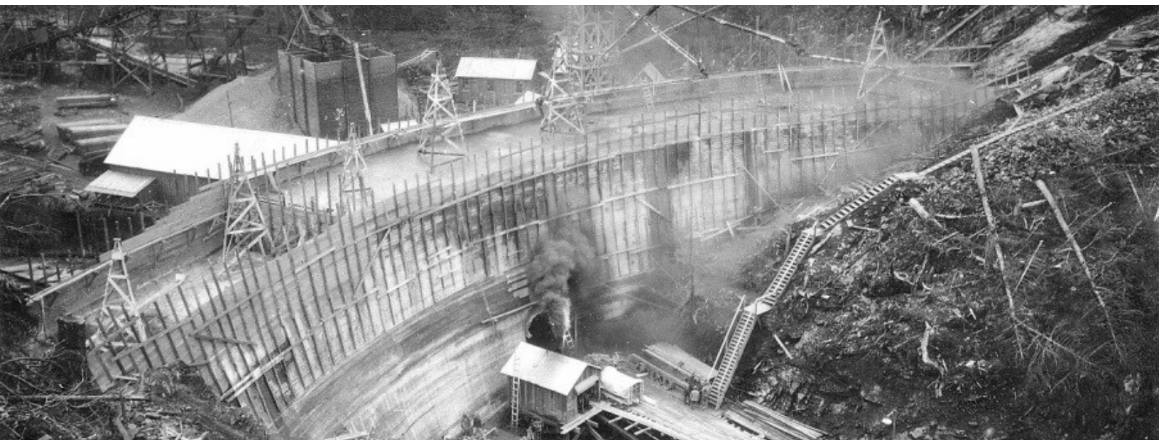
Salmon Creek Dam, Juneau, Alaska
