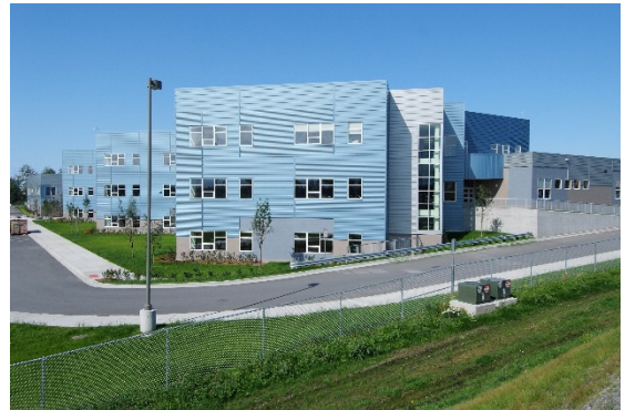
PND worked with McCool Carlson Green architects to provide structural design for the Clark Middle School addition and renovation project.
