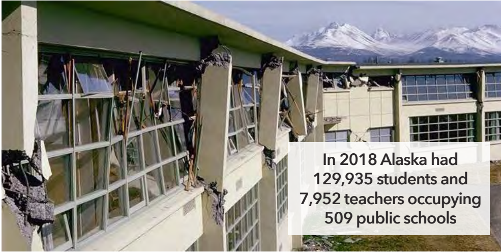
Concrete column failure at West High School in Anchorage, Alaska, after the 1964 Great Alaska Earthquake.
